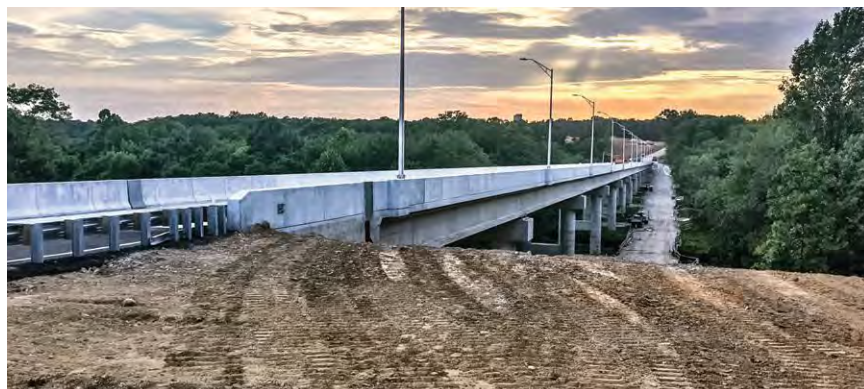
A new 11-span bridge provides a critical link to the Chesterfield Power Station.
